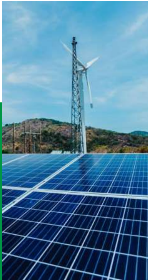
Solar Power EPC
